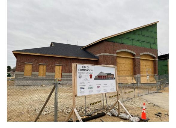
Progress continues on Phase I of the new Fire Station project with completion of exterior masonry work. Interior mechanical, electrical, and plumbing activity is on-going
