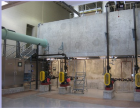
View of the hydrocyclones from atop the Actiflo system (above) and the front of the system from the process floor (below)
