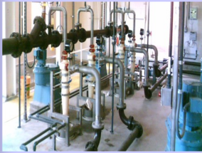
View of the hydrocyclones from atop the Actiflo system (above) and the front of the system from the process floor (below)
